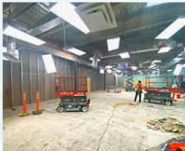
The back wall of the Auditorium has been removed and work is taking place behind a temporary wall, creating the area where hundreds of additional seats will be added. These areas will have operable walls that can be moved into place to allow these areas to be used for LIFE Groups and other meetings during the week.
